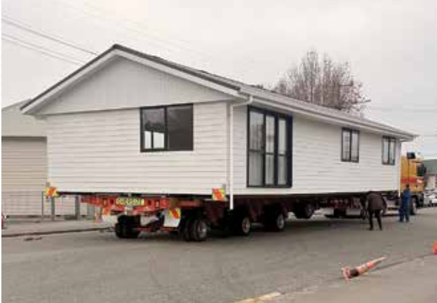
Our builders carefully prepare the house before moving it into position.
