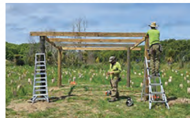
Kaimahi work on the new Hut and the roof, to host wānanga.
