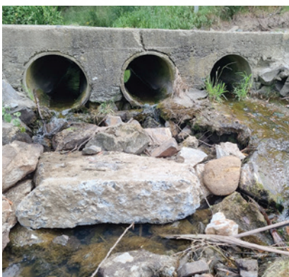
Downstream view of the Brooklands Road ford, showing poor fish passage characteristics present before construction of the rock ramp.
