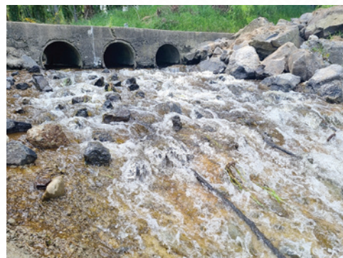
The Brooklands Road under high flows following the construction of the rock ramp.
