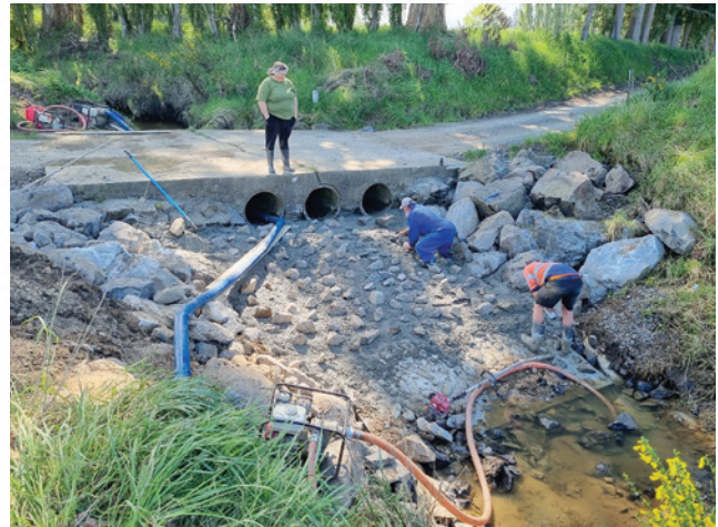
Above: Construction of the Brooklands Road rock ramp, showing the low gradient ramps with rocks placed to reduce water velocity and provide resting areas for fish.
