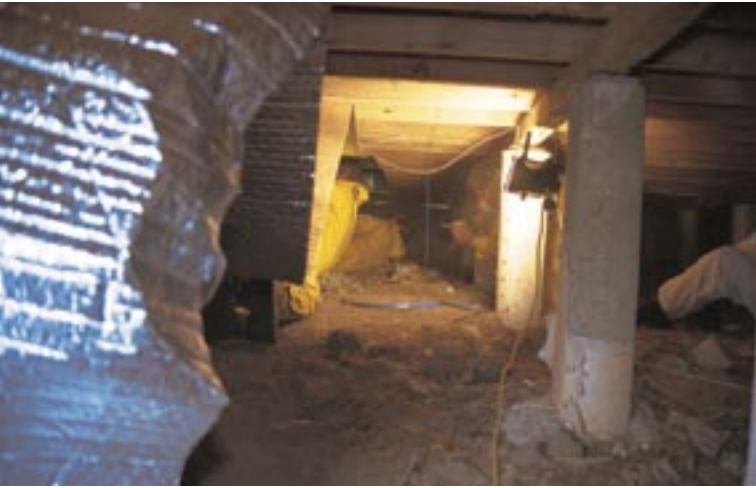
Installation at the home of Ann-Marie Ryan (mother of Kiri Bristow) – top: Grant Dunford helping with insulation blanket for the ceiling; above: Air Cell underfloor insulation going under the house.
